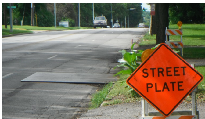
Exhibit 1: Example of a Street Plate in Place
